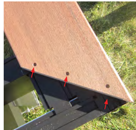
Within 1/2" of ends, along miters, and butt-joints
