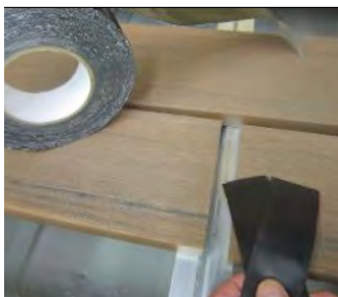
Self adhering TimberTech Pro-Tac Joist tape.
