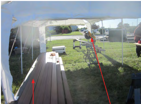
Decking stored flat and in shade—out of direct sun.
