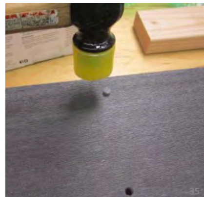
Tap plug 'flush' using a PLASTIC Mallet.
